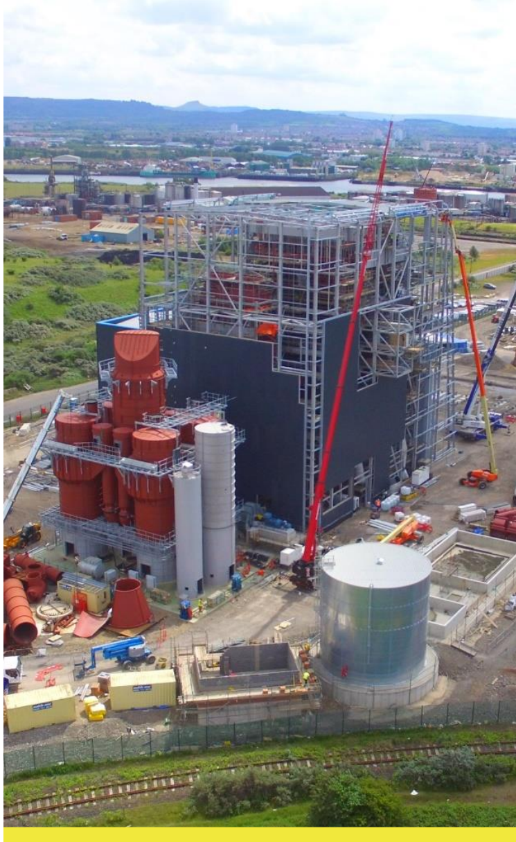
Above: Teesside Renewable Energy Plant 2,500 tonnes
